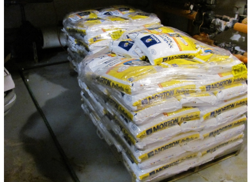
Softener Regeneration Salt Pellets Palletized 40 lb bags Consumed 400-800 lb/day
