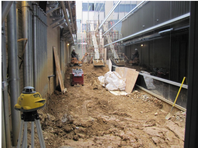
Stone & Soil Excavation
