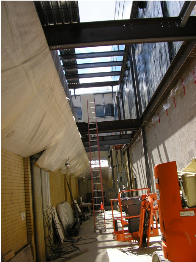
Building Structure Construction
