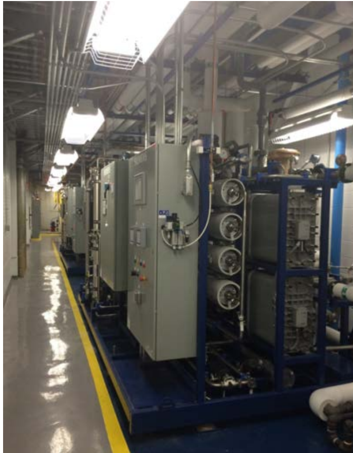
1 st Floor Dual RO Skids
