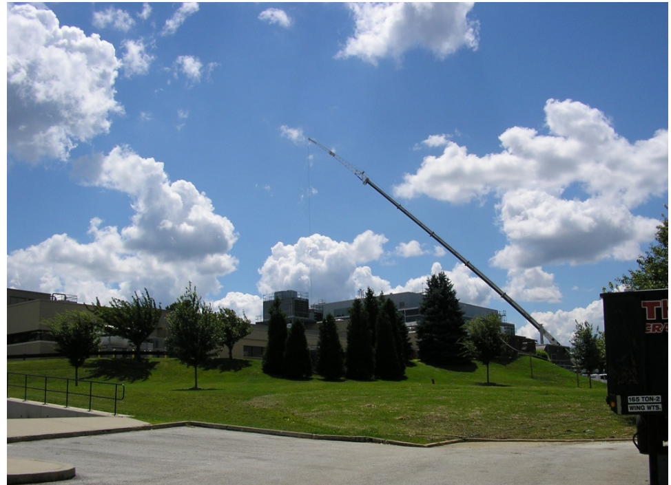
Large Crane due to Limited Access
