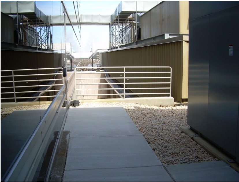
Top of Courtyard Looking NORTH
