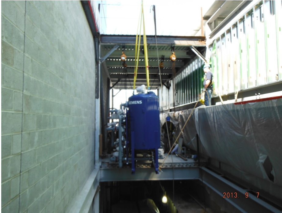
Installation of HPW Equipment
