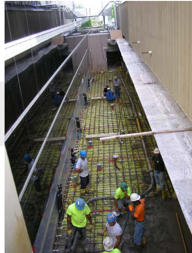
1st Floor Slab Installation
