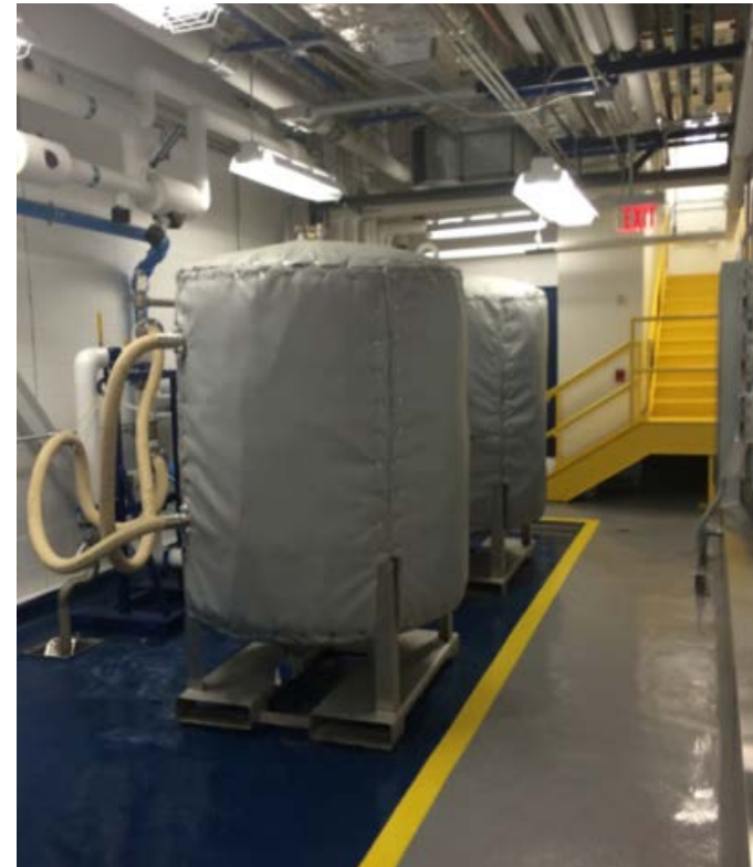
2 nd Floor Dual Carbon Filters
